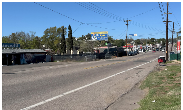
Existing roadway condition along Campo Road
