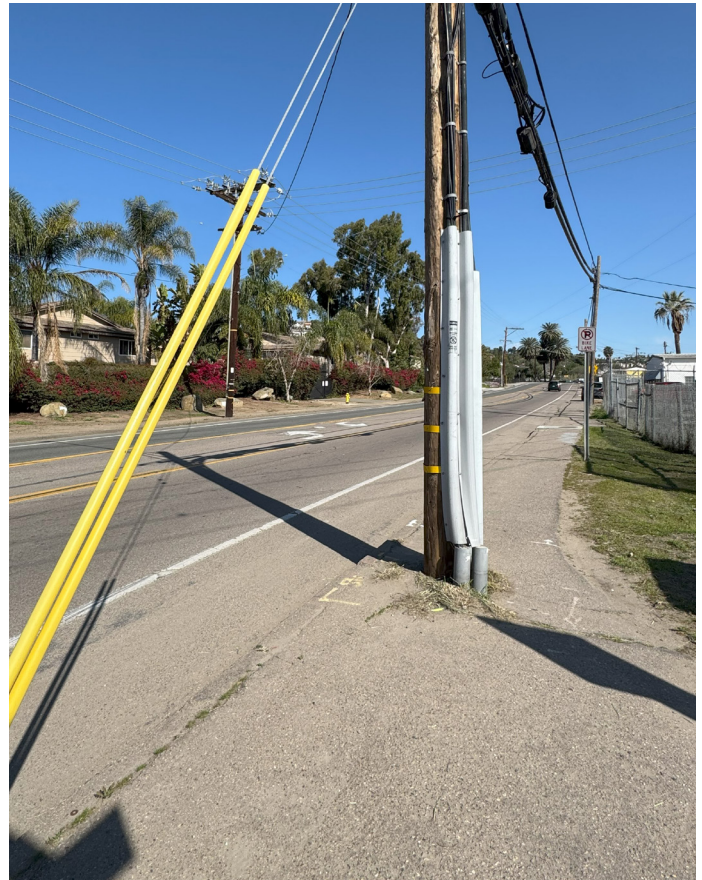
Utility poles in the middle of the pedestrian path of travel
