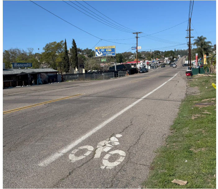
Class II bike lane on Campo Road (near Bancroft Drive)
